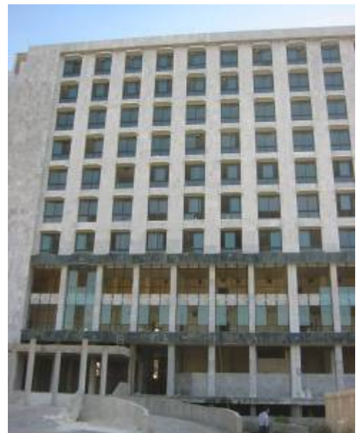
MOI HQ Building under construction
