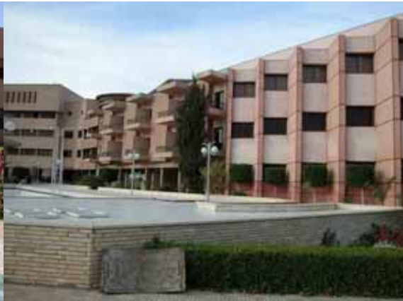
RCTWS accommodation building (right)
