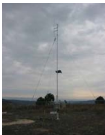
Automatic Weather Station (Nov.16 Dam, GDCB)
