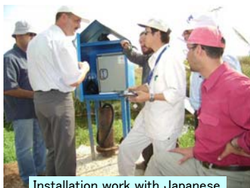
Installation work with Japanese Experts in GDCB
